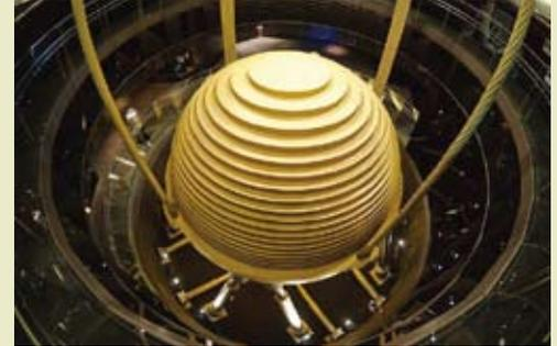
The 660 tonnes pendulum used in Taipei 101's major tuned mass damper (photographed by Armand du Plessis).
