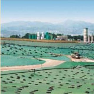
The landfill gas plant in the North-East New Territories Landfill at Ta Kwu Ling. The plant is expected to supply over 10,000 m<sup>3</sup>/hr of methane in 2015. (Courtesy of Hong Kong and China Gas Co. Ltd.)
