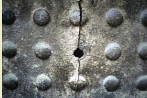
Cracks emerging from a rivet hole which can be found in many metallic structures. (© Petr Kastorsky | Dreamstime.com)
