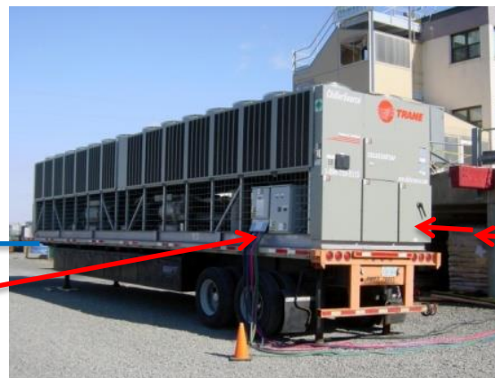
Mobile air-cooled water chiller
